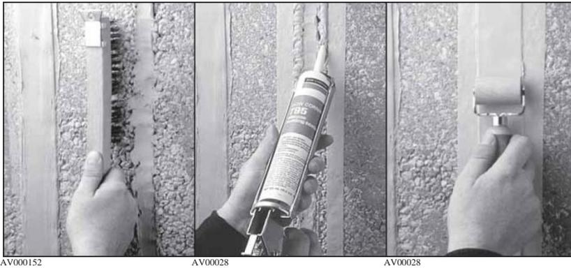
*Dow Corning 123 Silicone Seal is easily applied: prepare the substrate around the failed sealant; apply Dow Corning 795 Silicone Building Sealant; and apply Dow Corning 123 Silicone Seal.*
